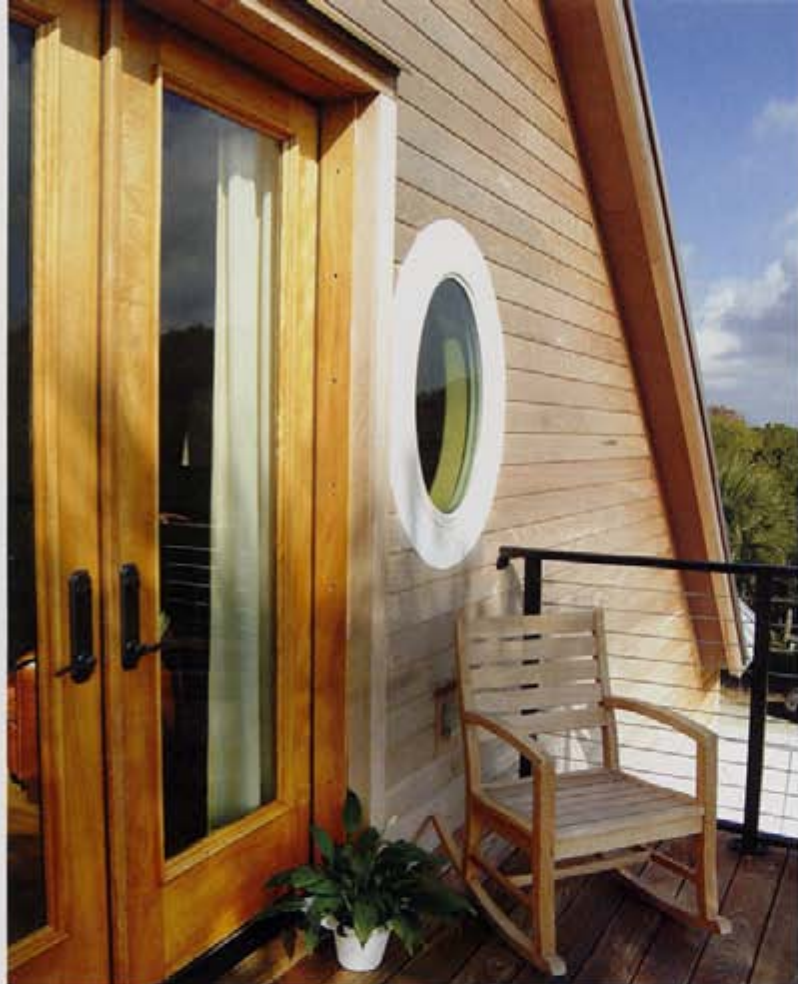
Above: The Bird House's old-fashioned porch is made of indestructible ipe lumber. Above left: Like its sister residence, the 1,530-square-foot Tree House features a variety of custom-fitted woods.
